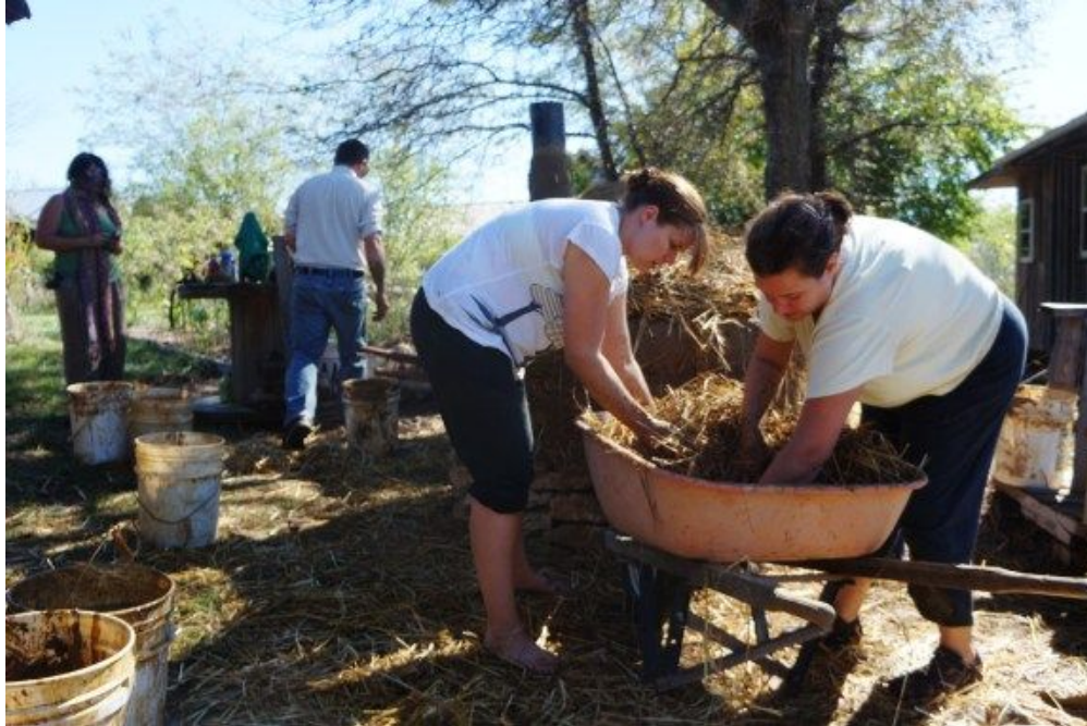
Tossing up some 'light clay straw' insulation in a wheelbarrow
