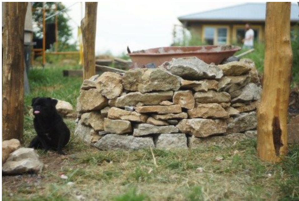
The start of a simple dry stack stone foundation
