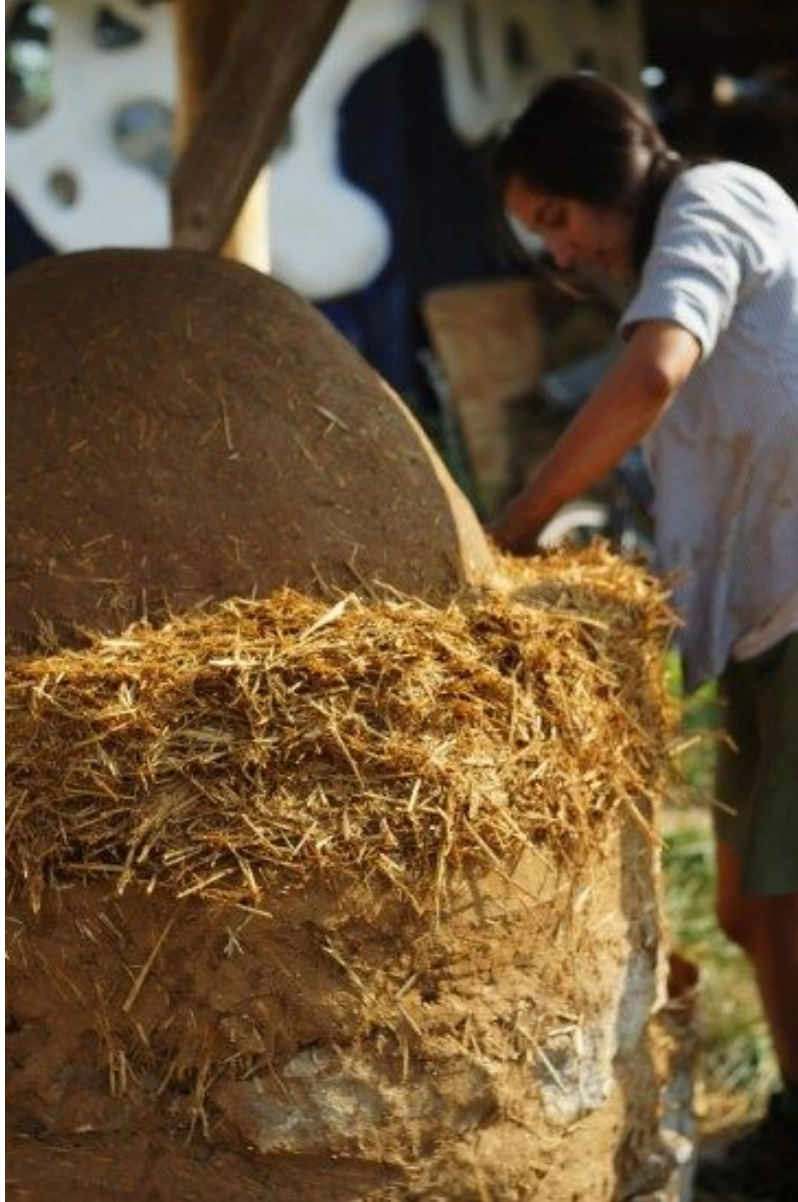
Building up the 'light clay straw' insulation
