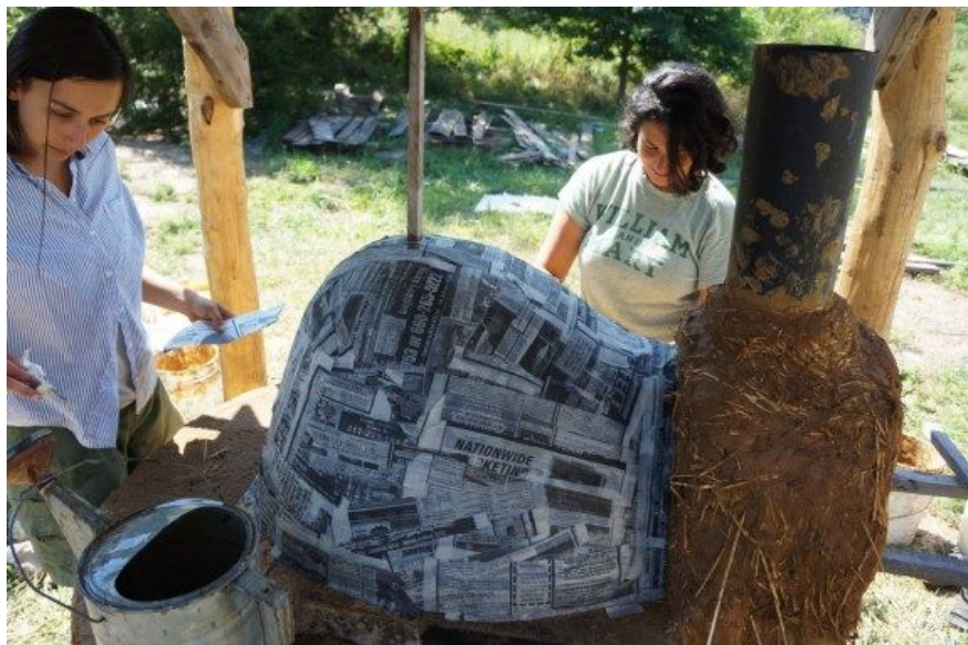
Wet newspaper is a good barrier between the sand form and cob
