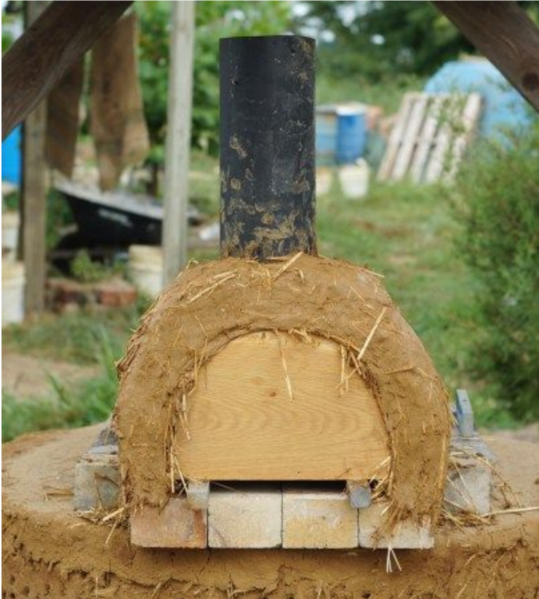
A roughly finished cob arch with stove pipe freshly installed
