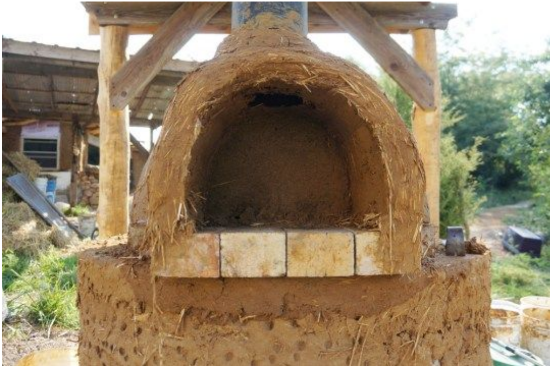
The doorway template is removed... and it's time to scoop out sand!
