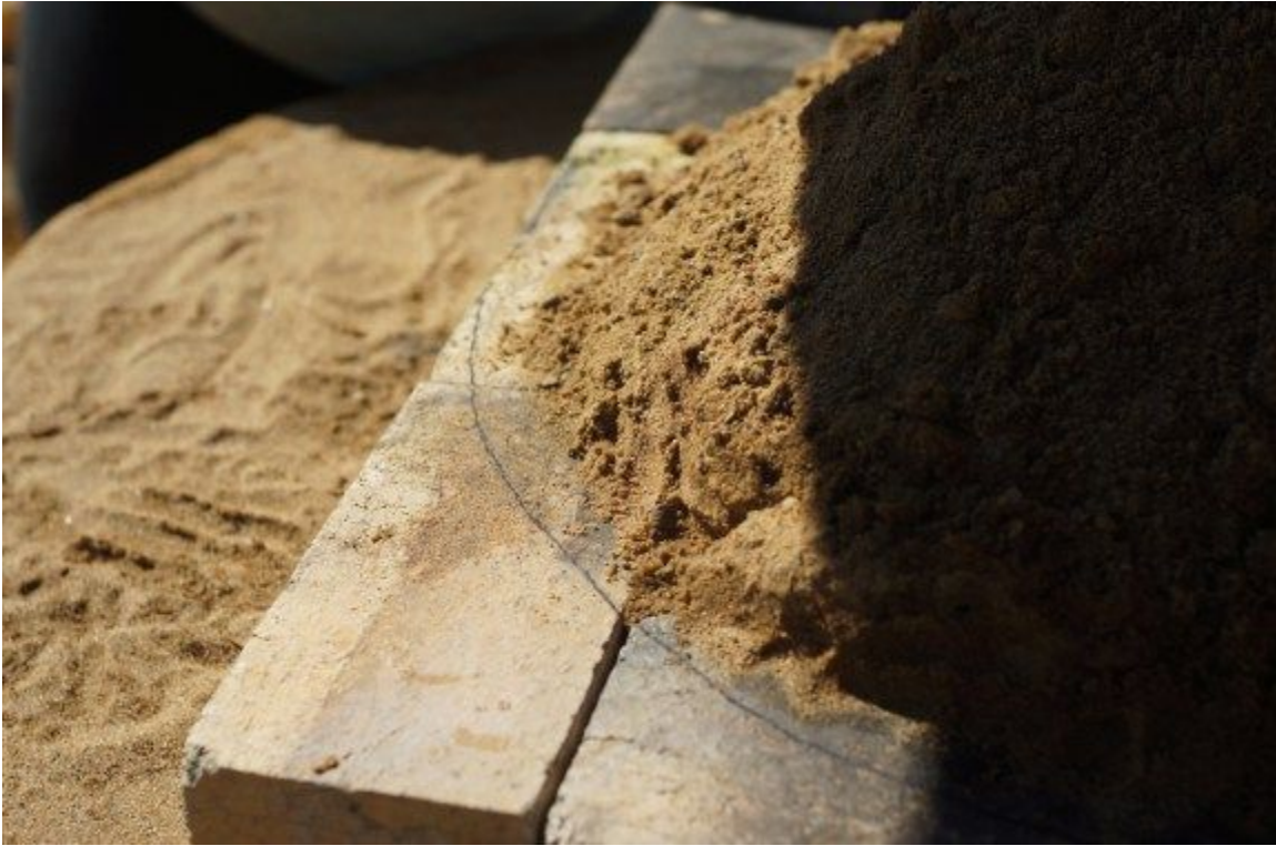
A 27" diameter circle is drawn out on the fire brick
