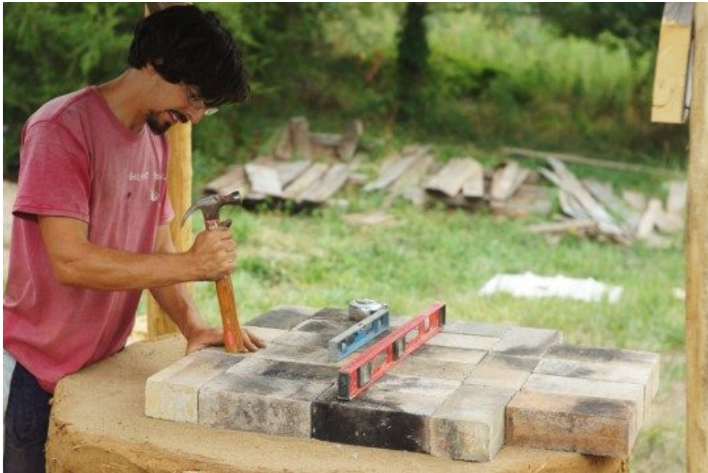
Setting the firebrick for the hearth, ensuring a level surface
