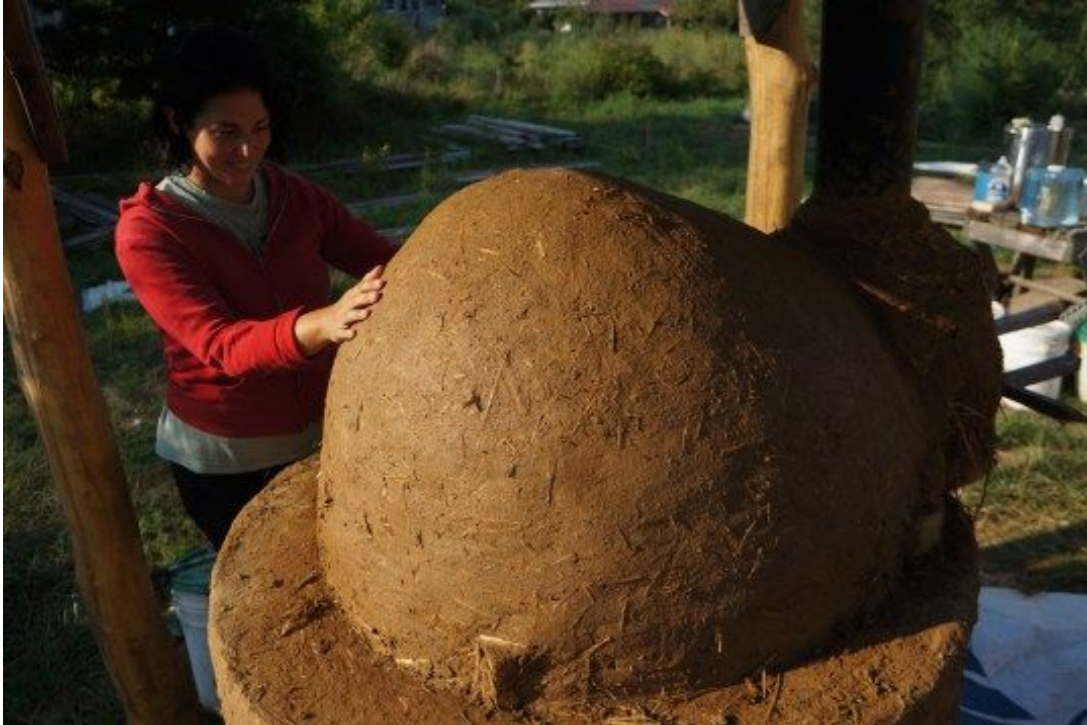
A 4" thick cob dome gets built around the sand form
