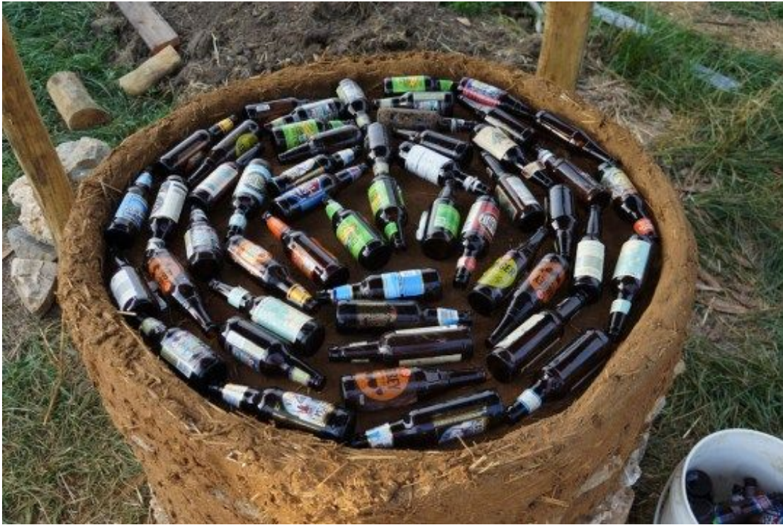
Beer bottles make for a very cheap method of insulating the firebrick hearth
