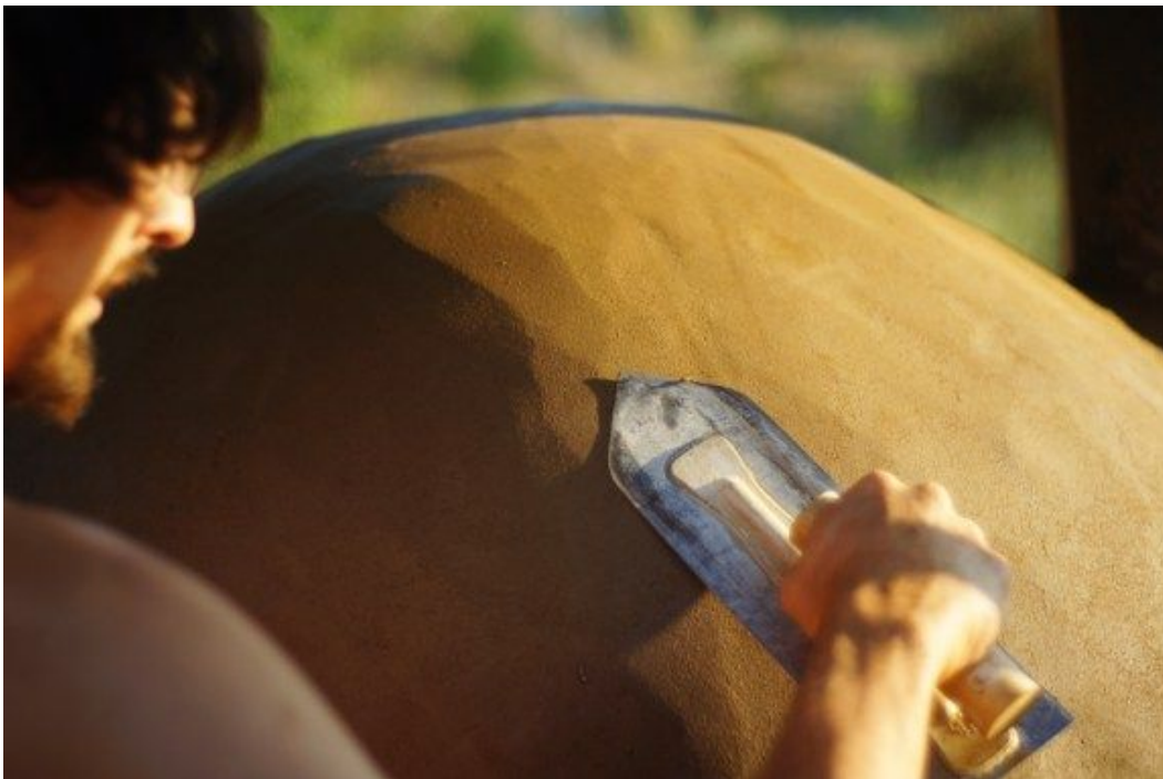
Applying finish clay plaster with a Japanese plaster trowel
